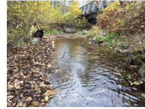
Trozzo Creek: downstream
